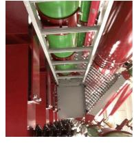
For the safety of the operator, our impulse generators are equipped with 3 points pneumatic earthing system to place to the earth the HV terminal of each capacitor and its tank. With this solution each capacitor is short-circuited and connected to the earth.
